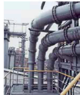
Fly ash pipes are among the plant components that are particularly endangered by wear. Kalenborn offers a variety of materials to ensure optimal service lifetimes: ABRESIST fused cast basalt, KALCOR zirconium corundum and KALOCER high alumina ceramics.
