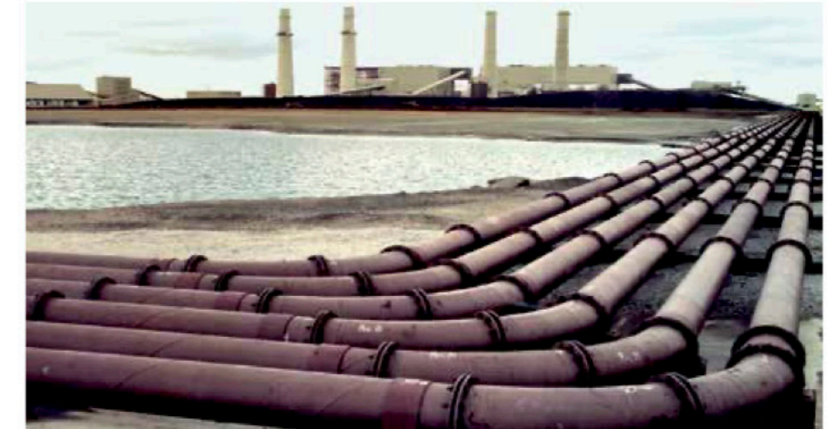
Wet ash pipe in North America; the pipes are flanged together.
