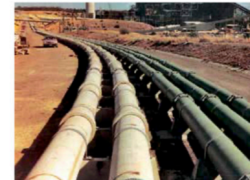
Wet ash pipe in North America; the pipes are flanged together.
