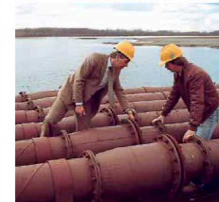
Long pipes require the use of expansion joints for linear extension.
