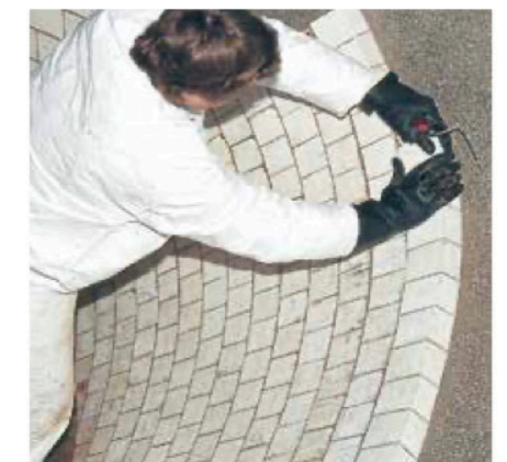
Kalenborn service solves wear problems on site
