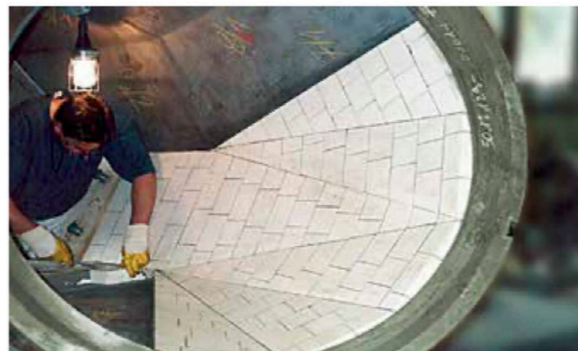
Octagonal hopper with KALOCER lining; for optimal adaptation the 50 mm thick shaped elements have been cut three-dimensionally
