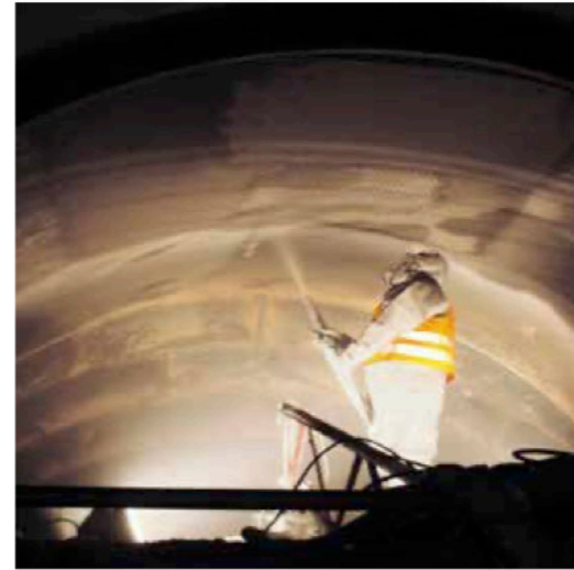
Protection of raw meal pipes against abrasive wear with hard compound KALCRET, lining thickness 25 - 40 mm, operating temperature 200 °C / 392 °F
