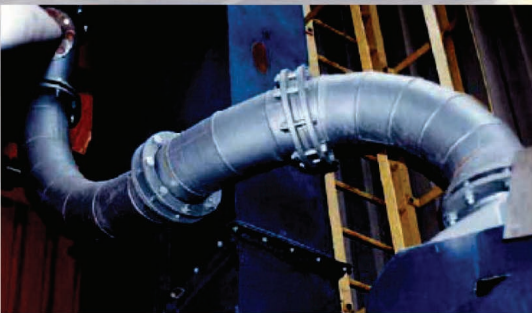
ABRESIST pipes and pipe bends protect against abrasion and corrosion
