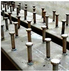
SHEAR CONNECTOR STUDS
