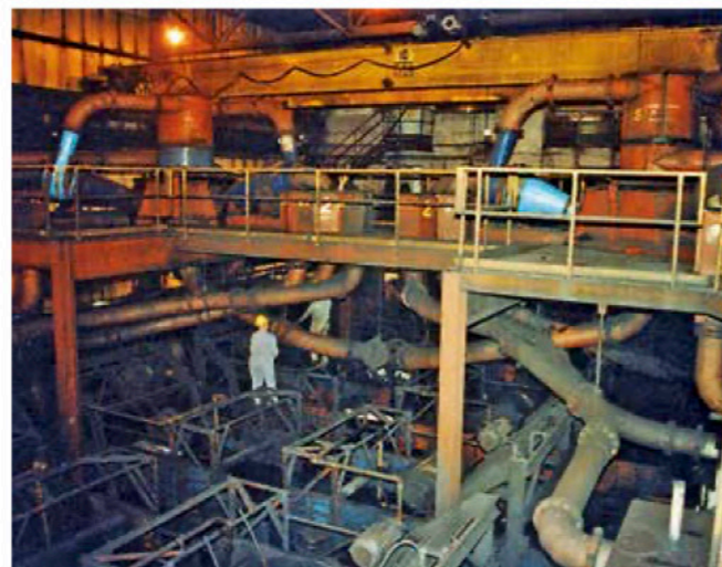
Hydraulic conveying pipes integrated in a coal preparation plant in North America. The pipes have been lined with ABRESIST. In this case they reach service cycles of more than 20 years.
