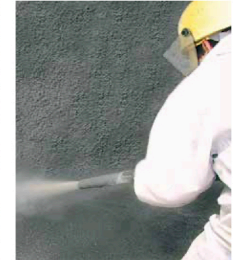
Kalenborn service solves wear problems on site
