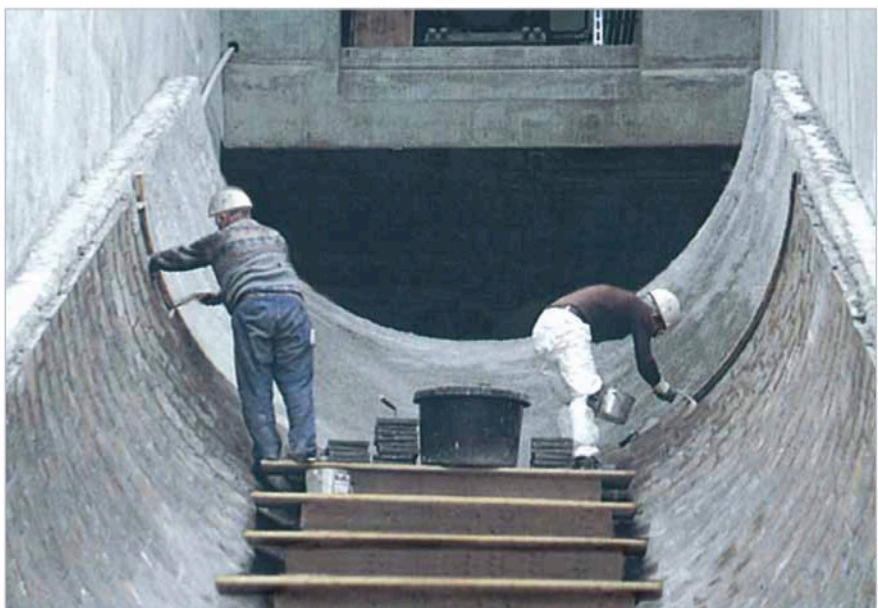
Quite often screw-type elevators are used for transport in waste water treatment plants. Continued proper functioning of the annular gap requires its being protected against wear. ABRESIST is successfully used for that purpose even at diameters of 3,000 mm and 15,000 mm length.
