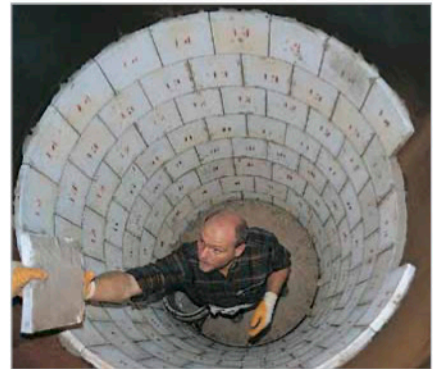
Potassium silicate based mortars are used in case of high thermal stress
