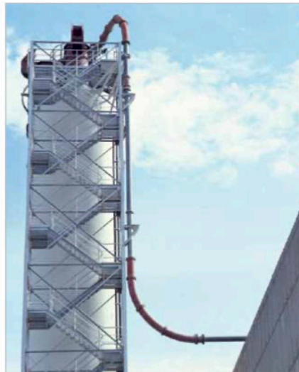
The bends and straight extension sections of the feed pipes to cement silos have been lined with ABRESIST
