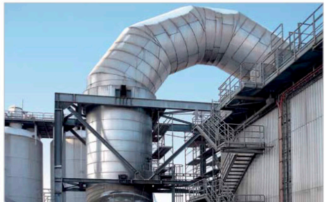
Sinter dust transport pipe in a German cement plant
