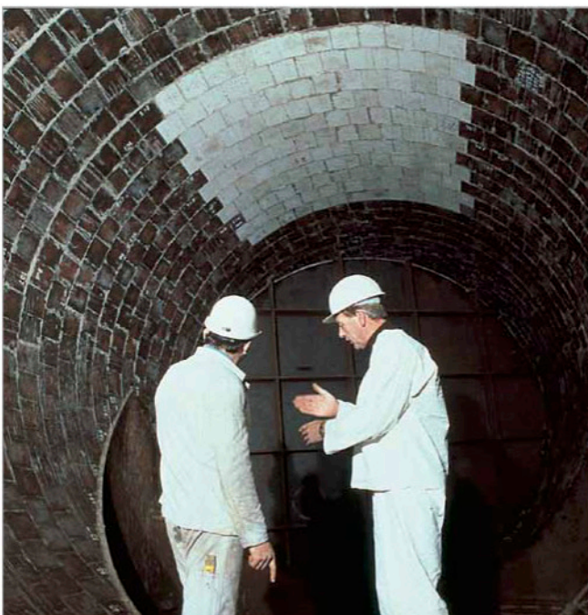
Abrasive sinter particles impinge on the KALCOR lining at 250 °C / 482 °F and at high velocity – combined with ABRESIST results in an economical solution
