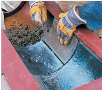
Setting in cement mortar
