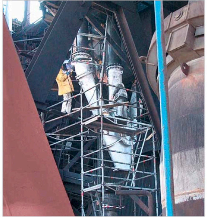
Pressure equalizing pipe set up near a blast furnace; the base metal has a thickness of 30 mm, the thickness of KALMETALL-W 100 hard overlay welding measures 6 mm; 450 mm diameter
