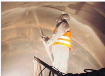
Overhead working possible without difficulty
