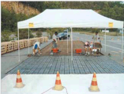
Fused cast basalt has performed well on automobile test tracks all over the world. Here, skid tiles are laid in Switzerland.
